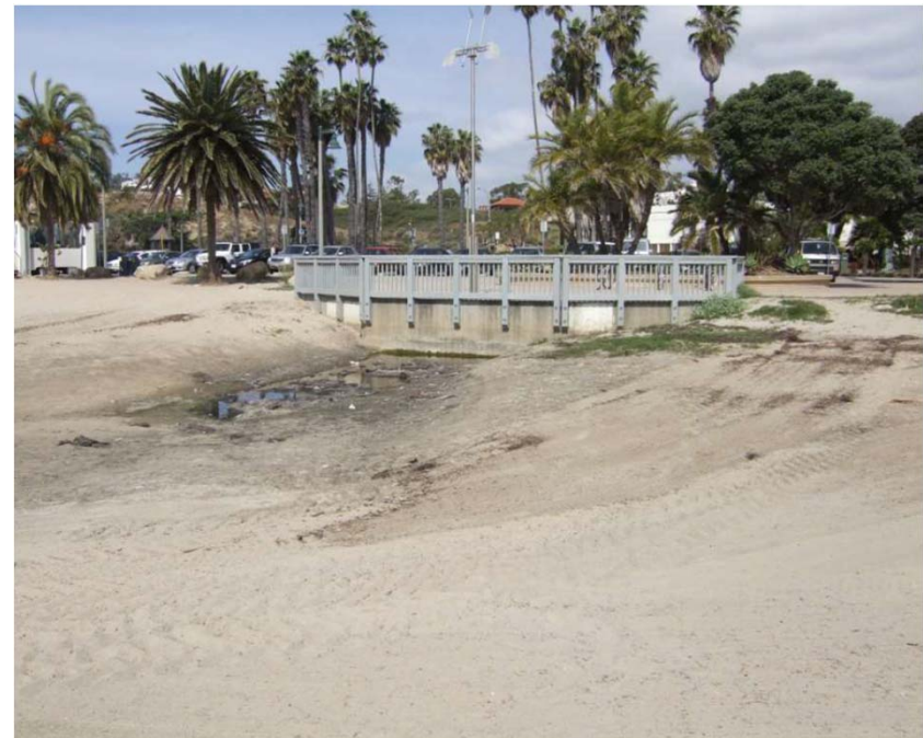
Honda Creek Culvert at Leadbetter Beach
